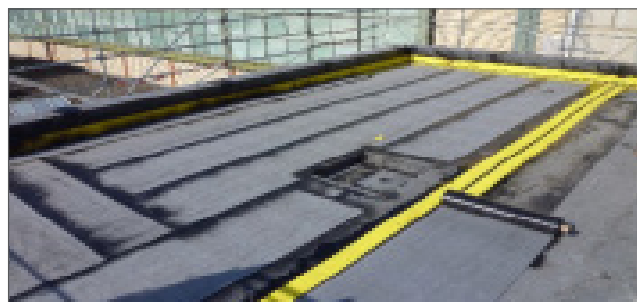
Simple sandwich installation between two geomembranes
